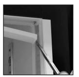
Remove silicone corner beads. Pry the screwdriver between plastic cover and cabinet frame. Pry from one end to the other.
