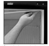
Snap plastic cover back to cabinet frame. Apply silicone at plastic cover corners.
